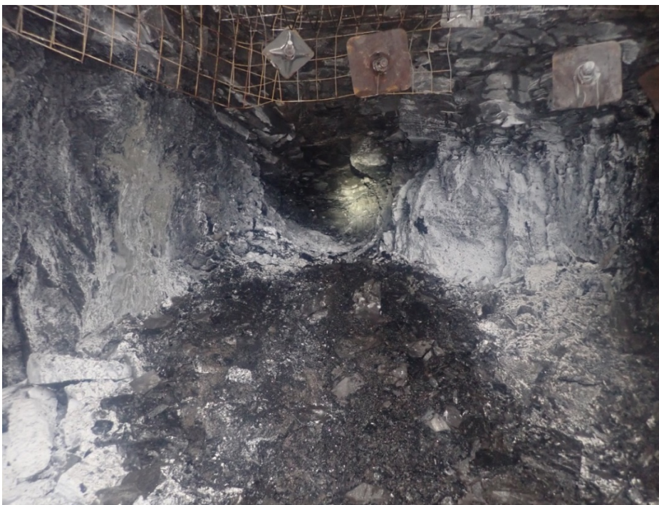
Figure 6: Event 3. View of left-hand side cone after strata support installed
