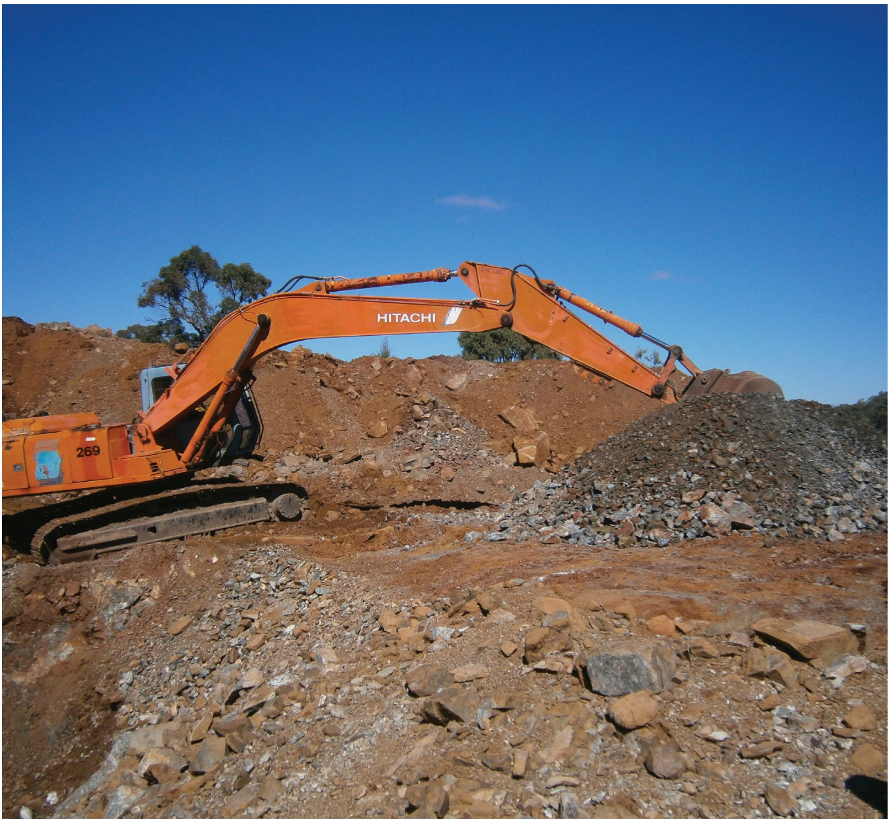
Extraction of rock sample for pilot plant
