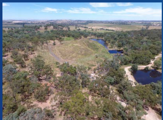
Kangiara Mine after remediation and rehabilitation works, December 2020
