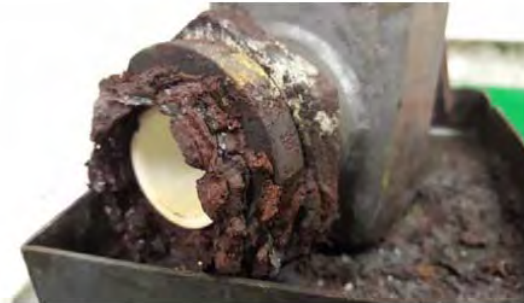
Figure 36. A photo of the gland after testing (Method 5) showing severe slurry leak and corrosion of the gland.
