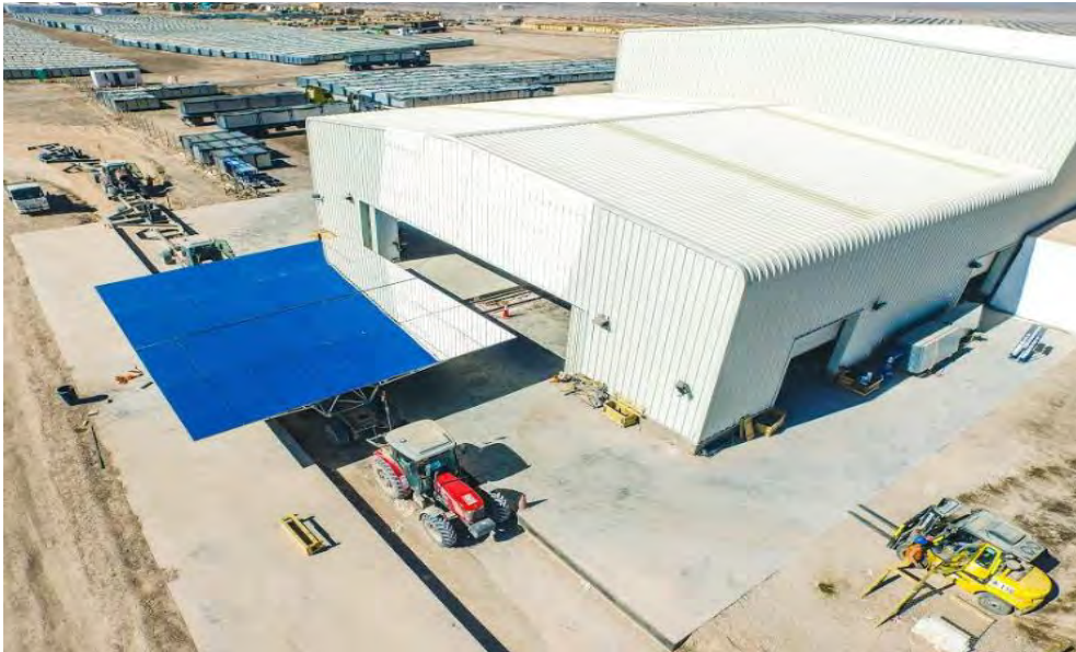
Figure 7. Manufactured heliostat being transported to solar field
