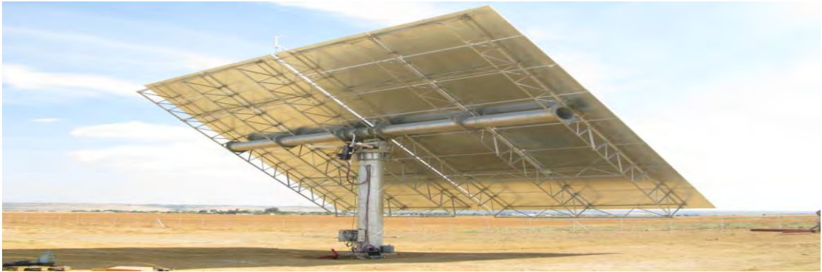
Figure 8. Heliostat installed in the solar field
