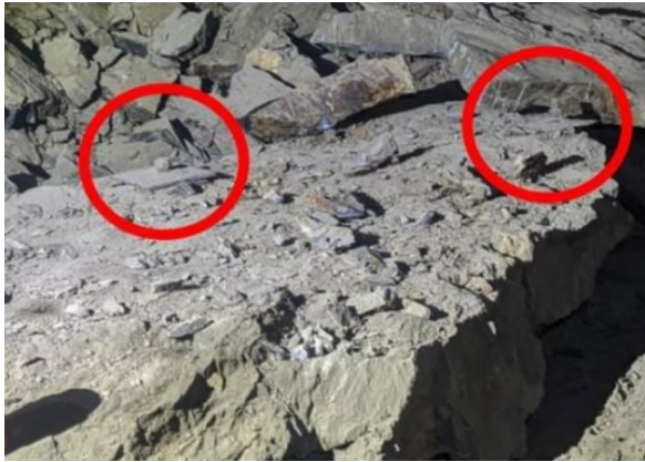
Below: Plates still in place.
