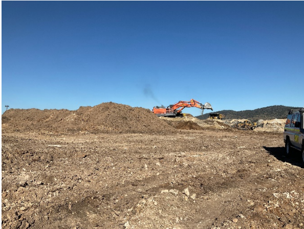
Figure 7. Clearing and topsoil stripping of the area of exploration drilling
